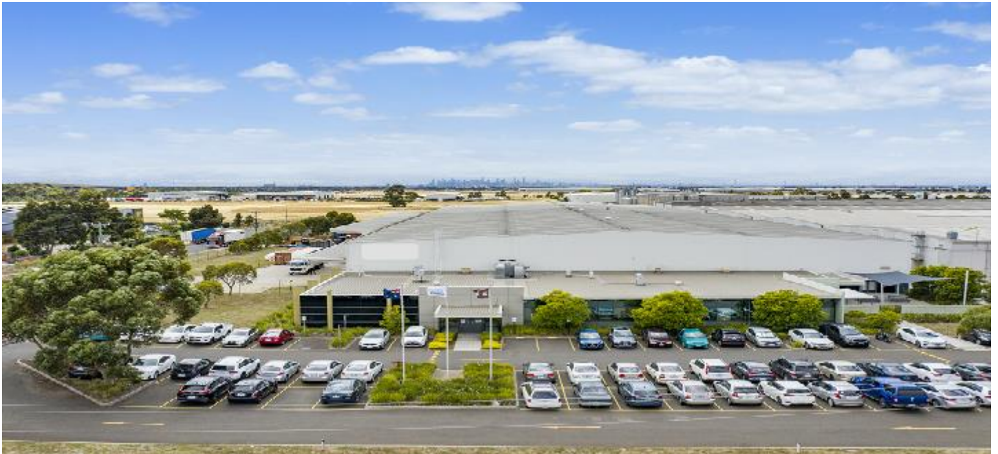
2-10 Bliss Court, Derrimut VIC
