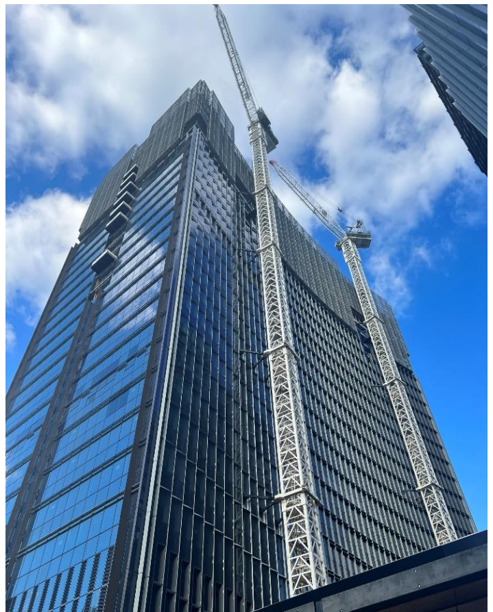
Melbourne Quarter Tower, nearing completion
